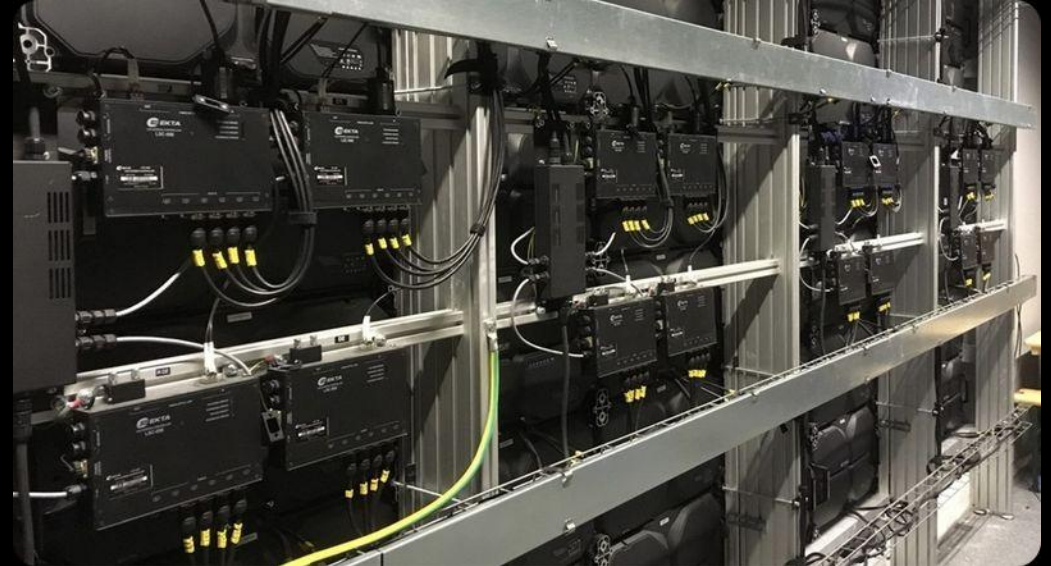
Power supplies, screen controllers and data cables behind the wall: work here only when isolated and by qualified staff.
